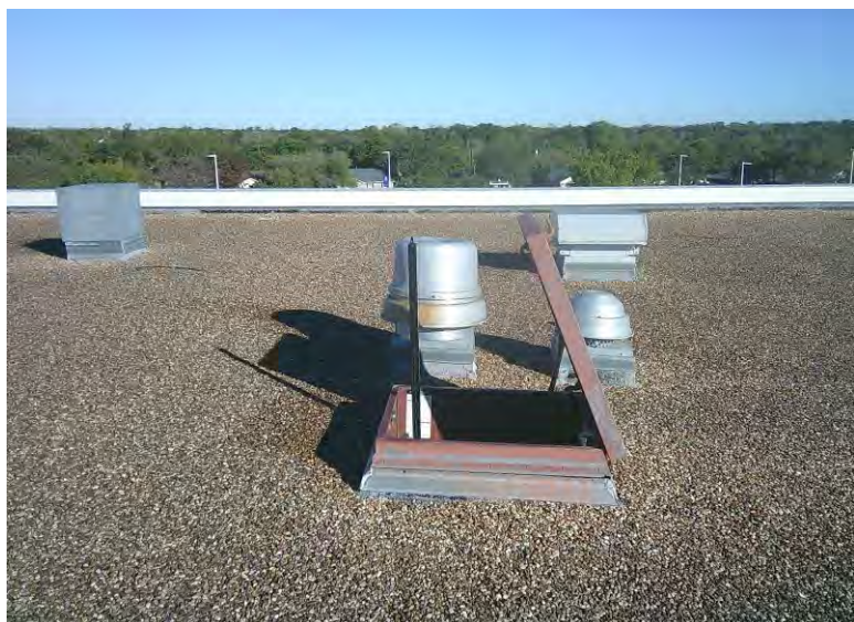
2. View of the Building F Roof
