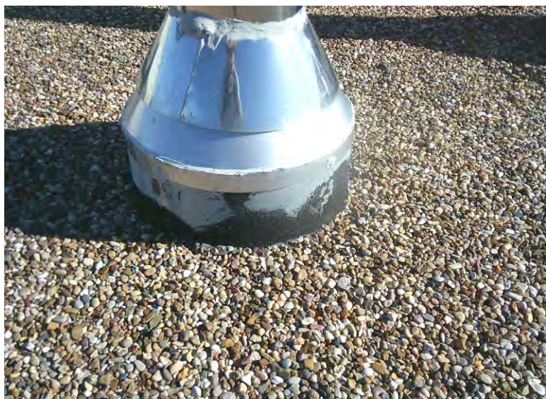
10. Asbestos Homogeneous Area 5 – Black roof tar; Sample 05
