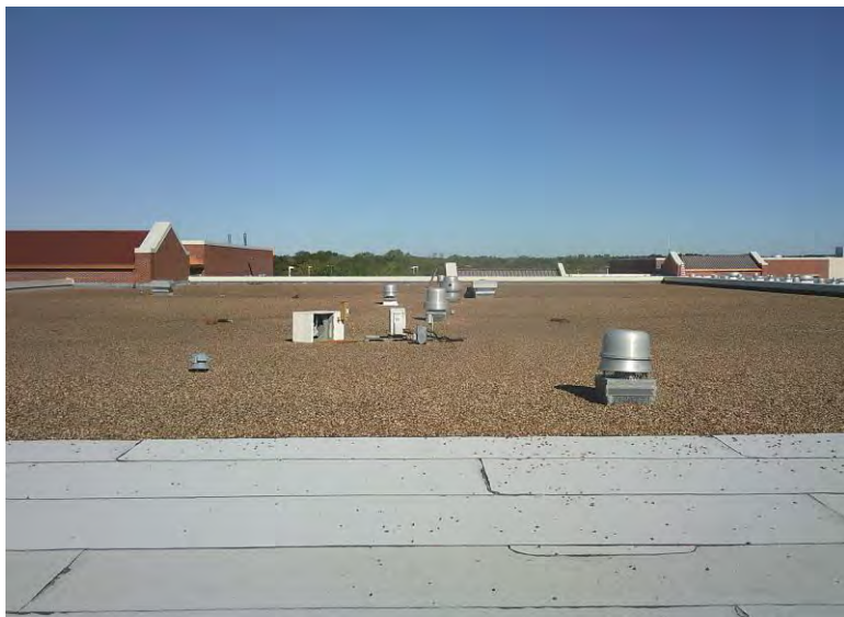
2. View of the Building H Roof
