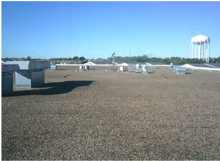
4. Another view of the Building F Roof
