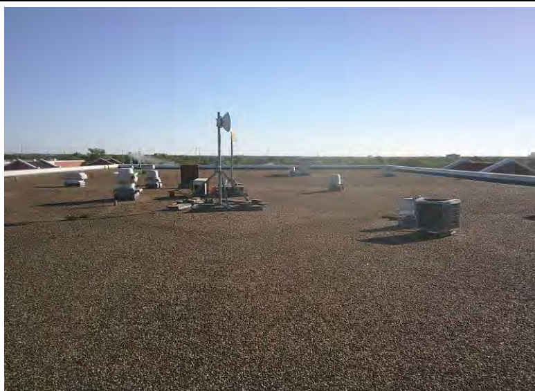
3. Another view of the Building F Roof
