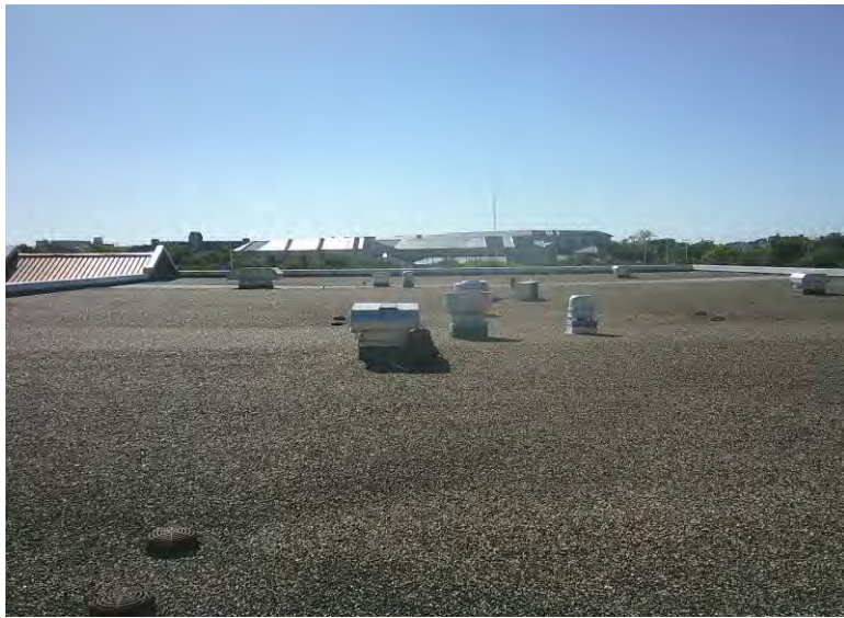
4. Another view of the Building H Roof
