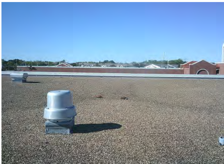
3. Another view of the Building H Roof
